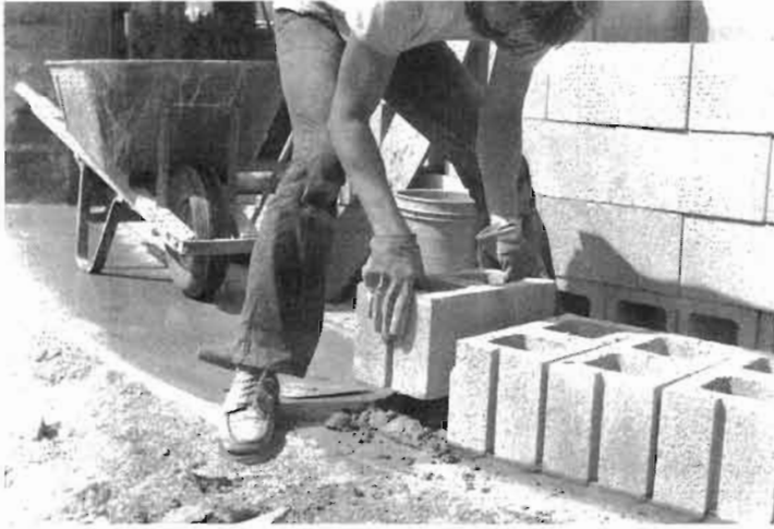
Fig. 5.10: Earthwood: the first course of 8" corner blocks is set in mortar.
