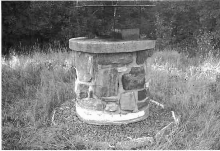
Fig. 11.3: Any projection through the earth roof – skylight, chimney, vent stack – should be surrounded by good drainage material, such as #2 crushed stone. out of plumb. Once again, bad drainage was the culprit. We solved the problem by carefully removing the topsoil next to the flashed retaining boards and replacing it with crushed stone, drained to the edge of the building. Even though you will see detailing in the literature for retaining boards at the roof edge, my strong feeling now is to leave them out in favor of either sods around the edge or treated retaining timbers supported by 1-inch pressure-treated shims. Both of these methods are described in Chapter 8. The exception would be steeper pitched roofs, such as Chris Dancey's, also in Chapter 8.
