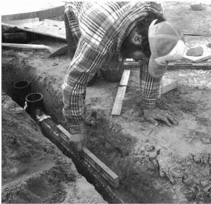
Fig. 4.10: Installation Tips for Underfloor Plumbing Dennis Lee checks the slope of the underfloor drains. Plan the plumbing so that all traps are accessible. In the case of a bathtub or shower on the first floor, this will usually necessitate “boxing out” a small area so that concrete cannot get in around the trap or drain. An 18-inch square box made of 2-by-6 material can be seen in Figure 4.9. It provides access to our shower drain and trap. Another good reason for the box is that – thanks to the ubiquitous Mr. Murphy of the famous law – it is very difficult to get the drain in exactly the right place with respect to adjacent walls, which are still non-existent at this point in time. Within the box, you can still make final adjustments to a drain location at the time of shower- or tub-base installation.
