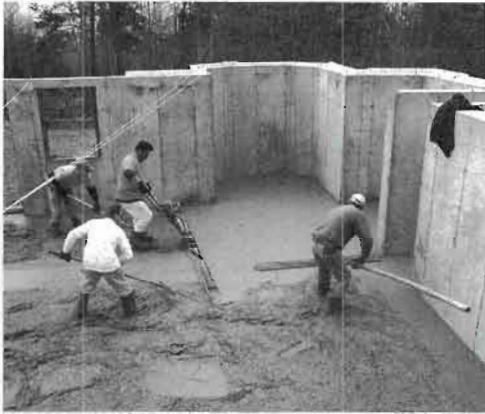
Fig. 4.15: One man operates the power screed while another bullfloats right behind him.
