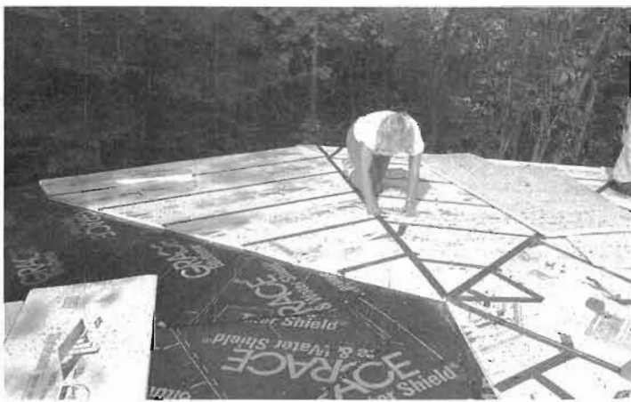
Fig. 8.2 (right): The author caulks the cut edge with Bituthene® Mastic.
