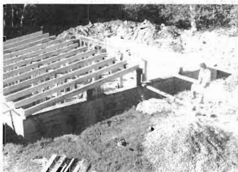
Fig. 6.9: Log End Cave, with half of the rafters in place.
