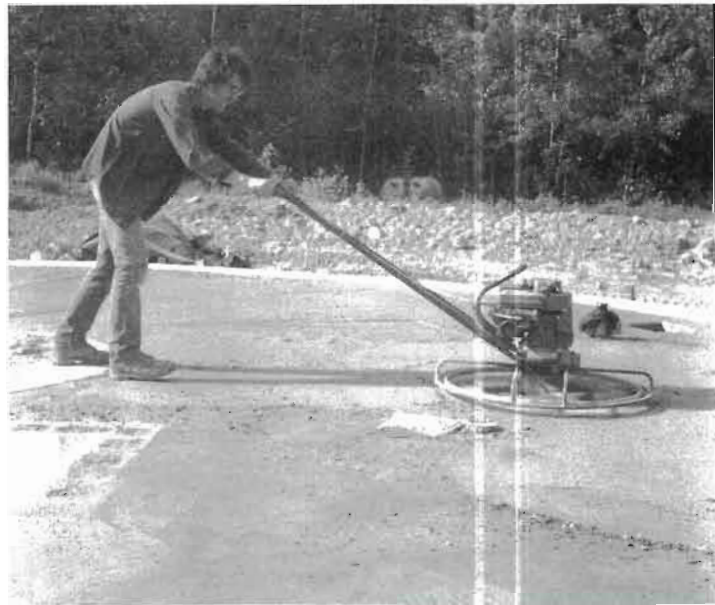
Fig. 4.17: Jonathan Cross power-trowels the slab at Earthwood.
