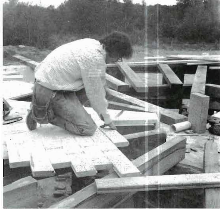
Fig. 6.17: Jonathan Cross nails the two-by-six planking to the radial floor joist system. Even short scraps are useful.
