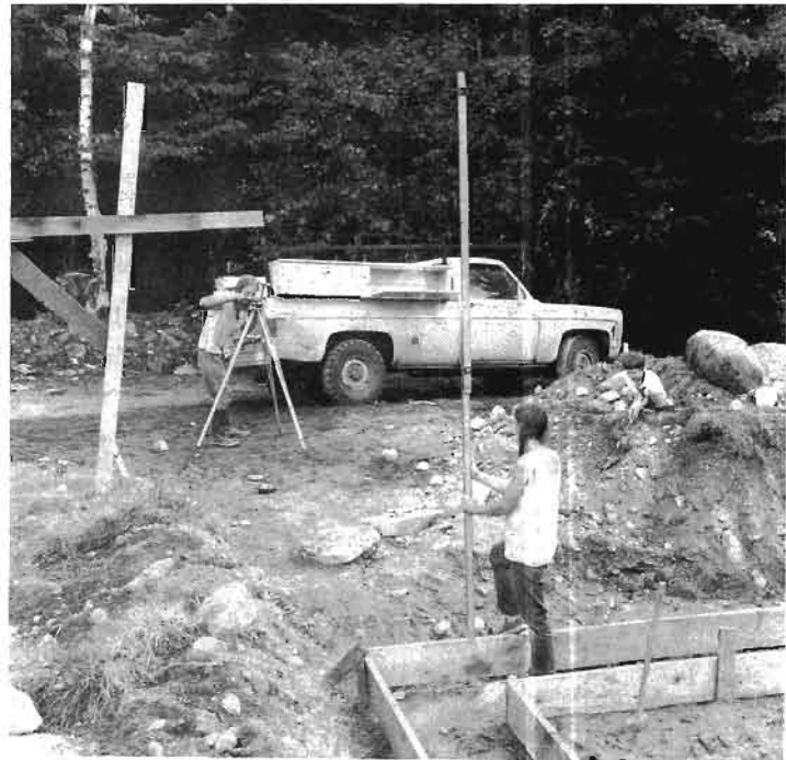
Fig. 3.11: Jaki holds a grade stake while a friend uses a contractor's level to assure that the inner and outer footing forms are all at the same grade.
