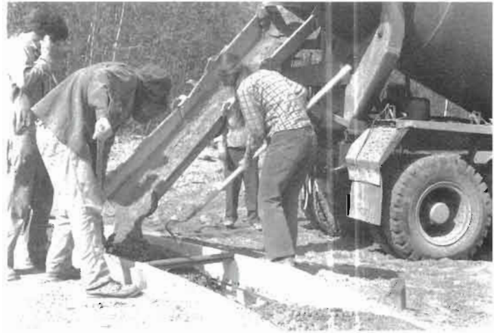
Fig. 3.22: Pouring the footings at Earthwood.
