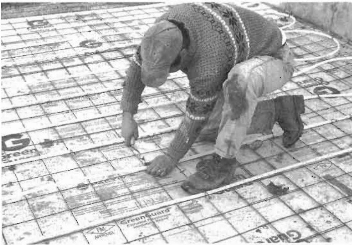
Fig. 4.6: Steve Bedard fastens his polyethylene tubing to the wire mesh with a special rotating hook made for twisting tie bands.
