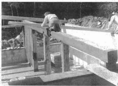
Fig. 6.8: We slide a rafter along the girders.
