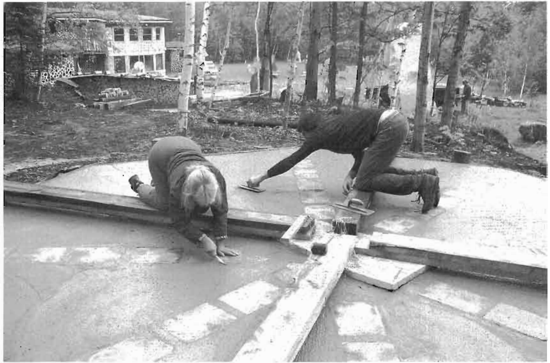
Fig. 10.4: Jaki points around slates set into the fresh concrete at Stoneview, while intern Nick Brown hand-trowels the triangular spaces between the eight slate "spokes."
