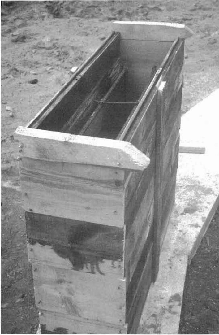
Fig. 4.16: We formed the buttresses with recycled 2 × 6" tongue-and-groove silo boards.
