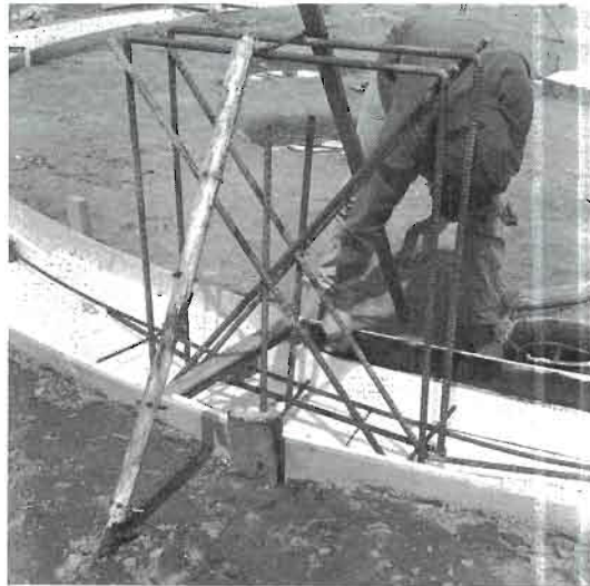
Fig. 3.19: At Earthwood, the buttress cage is made of #6 (3/4") rebar.
