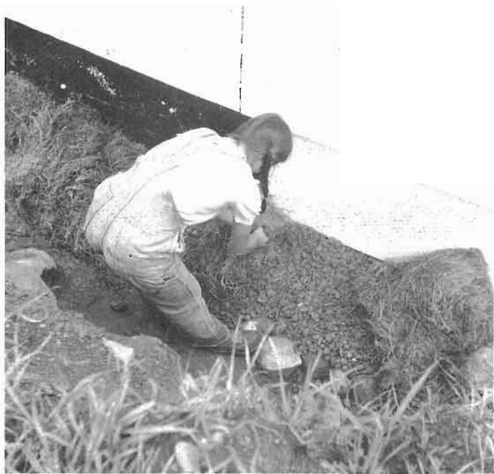
Fig. 7.15: Jaki spreads hay or straw on the crushed stone surrounding the drainage tubing.
