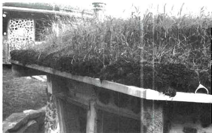
Fig. 8.18: Moss sods drain well, retain the earth and look natural. Note "half-pipe" for drainage.
