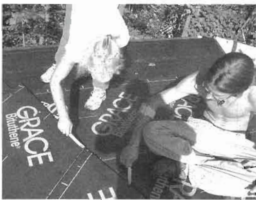
Fig. 8.3 (above): Jaki and Darin Roy feather the edge of the mastic with pointing knives, to approximate the factory edge of the Bituthene® membrane. The mastic stops the cut edge from raising up or "fish-mouthing."
