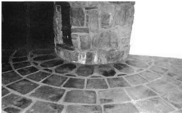
Fig. 10.5: The slate floor draws one's eye to the masonry stove at Earthwood's center.
