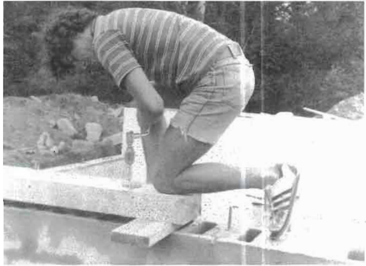
Fig. 5.13: Turn the plate over and drill holes through it of the same diameter as the bolts. See text for countersink procedure.
