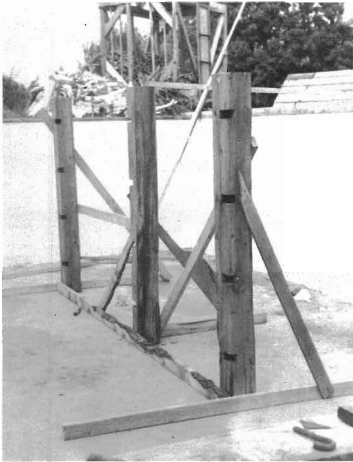
Fig. 6.4: nicely by itself, take it down and measure and mark the other end. You only get one try at the top end, so be careful. On the plus side, if it is a little off, the error can always be made up with wooden shingles. We temporarily braced the support posts for the main girders.
