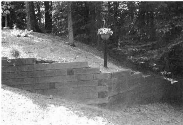
Fig. 9.5: This retaining wall is made of 6 × 6" pressure-treated timbers.
