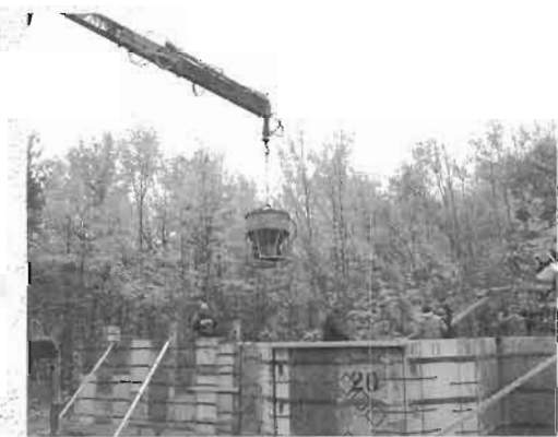
Fig. 5.1: Strong forms retain the concrete, which is delivered by chute, directly from the truck, or by hopper, controlled by the operator of the articulated boom.
